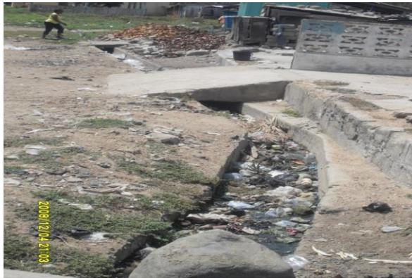
**Plate 6: A choked gutter**
